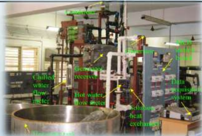
Absorber Refrigeration system
