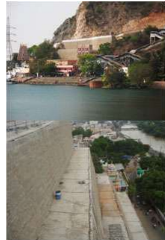
Construction of Very High Retaining Walls using Geosynthetics
