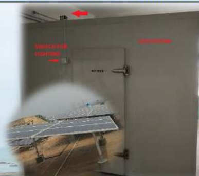
Solar Cold Storage
