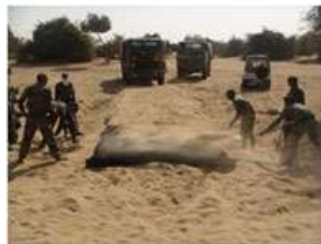
Construction of Expedient Road Bases
